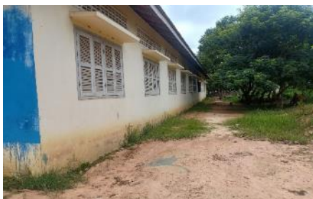
One of the concrete buildings at Srekvav High School
