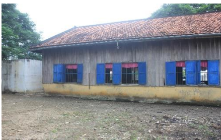
One of the buildings at Svaykang Primary School
